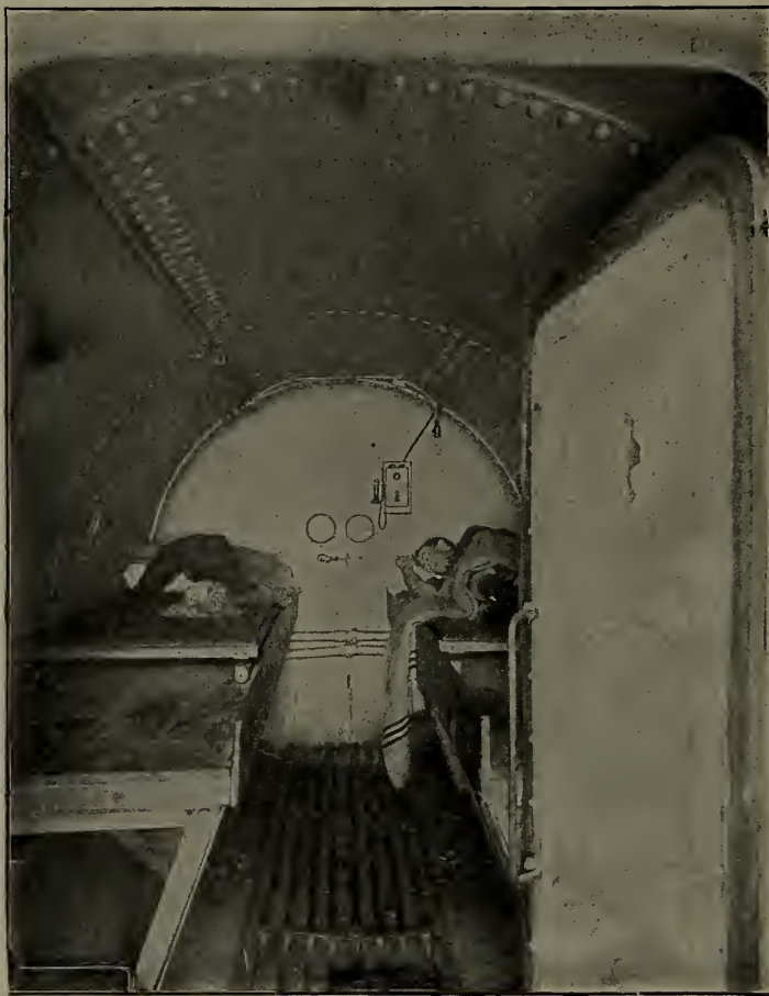
FIG. 1.—Interior of Medical Air Lock.
